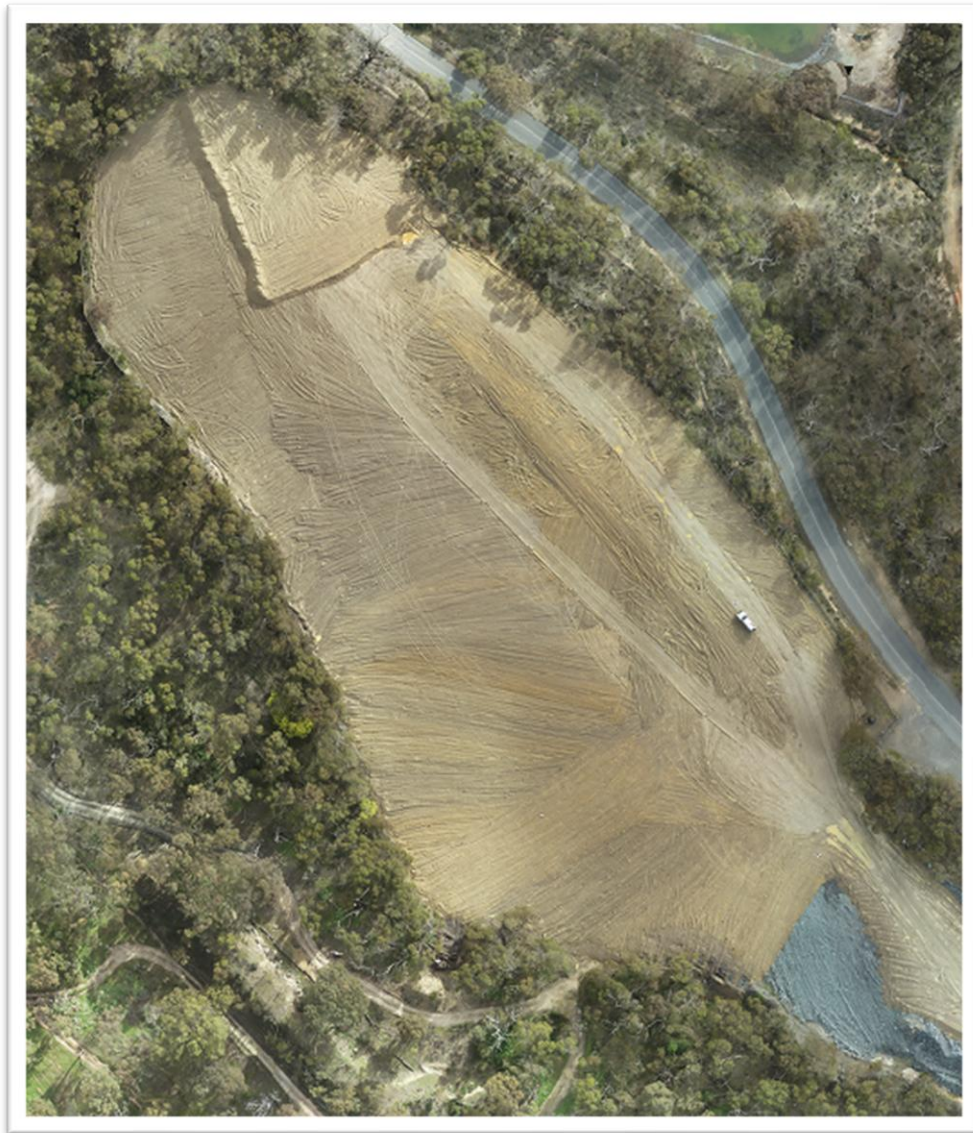
FIGURE 20 DAVIS PIT DURING 2022 SOIL WORKS
