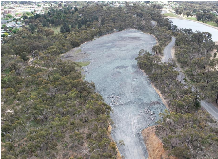
Figure 22 Davis Pit rockfill and landscaping
